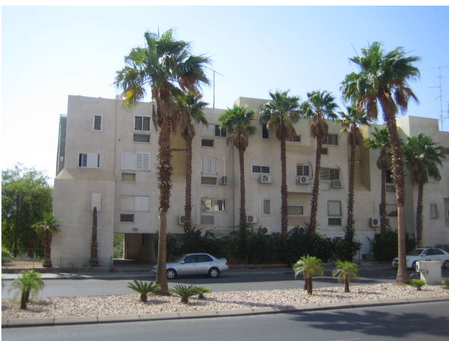
View of Apartment 1146 building on Sheshet HaYamim.
